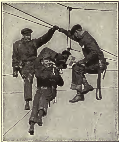
THE HAZARDOUS LIFE OF A RAILROAD LINEMAN
